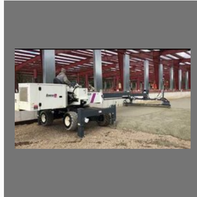
Laser Screed Concrete Flooring Services
