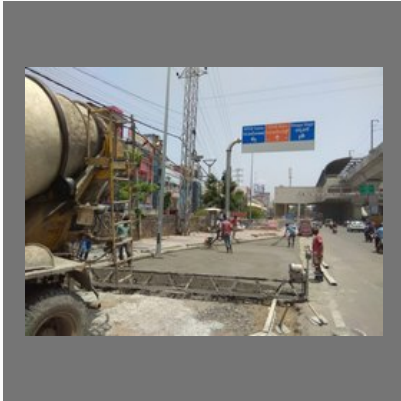
Truss Screeding Services
